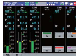
DIO operation monitor screen
